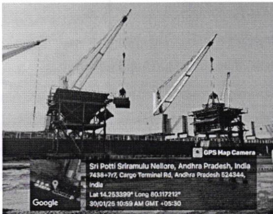
Mechanized system for loading of coal into dumpers
